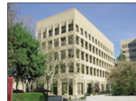
Keith Administration Building (KAM)
